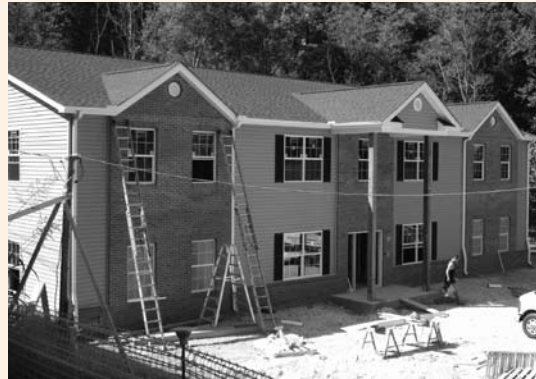
Construction of Apartments at Baker Avenue
